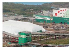
4. Production Unit (BKPRU-4) • potash producing plant (standard MOP) • potash mine, ore resources: 1,851 million tonnes 1
