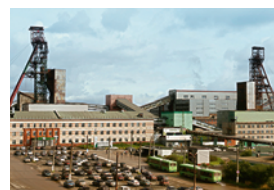
2. Production Unit (BKPRU-2) • potash producing plant (standard and granular MOP) • potash mine, ore resources: 318 million tonnes 1
